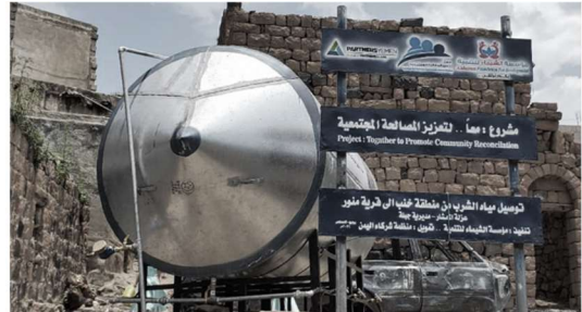
Water network collection point in Manwar village
