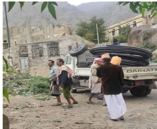
Installation of water network division room in Salah
